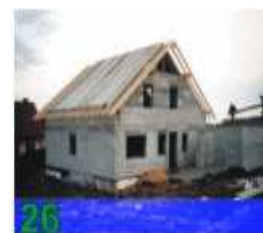
11. shell of house is finished after 14 days
