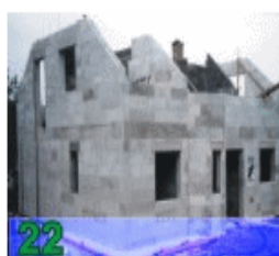
11. shell of house is finished after 14 days
