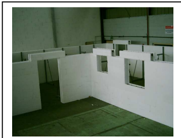
10. Fifth layer, lintels in place
