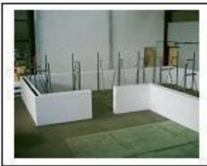
5. vertical alignment with trestles
