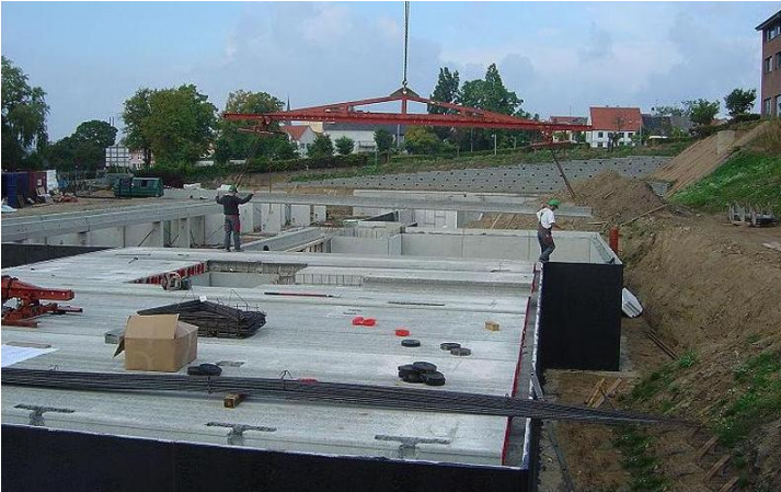
Prefabricated Hollow core slabs
