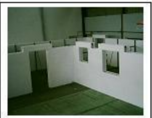
7. fifth layer, lintels in place
