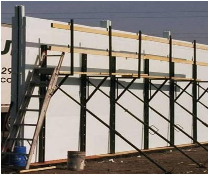
Wall alignment with braces
