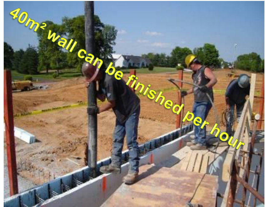
Pouring with Ready Mix concrete
